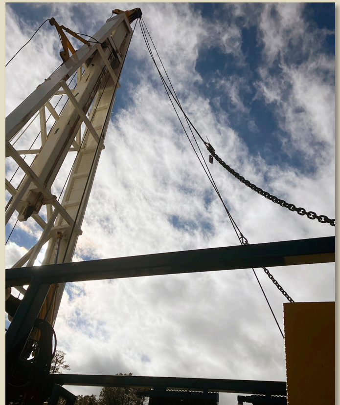
Well Mast Up Rig Inspection
